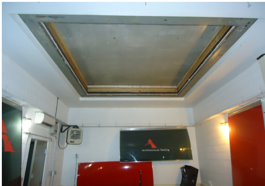
Receive Room View of Test Specimen Installation
