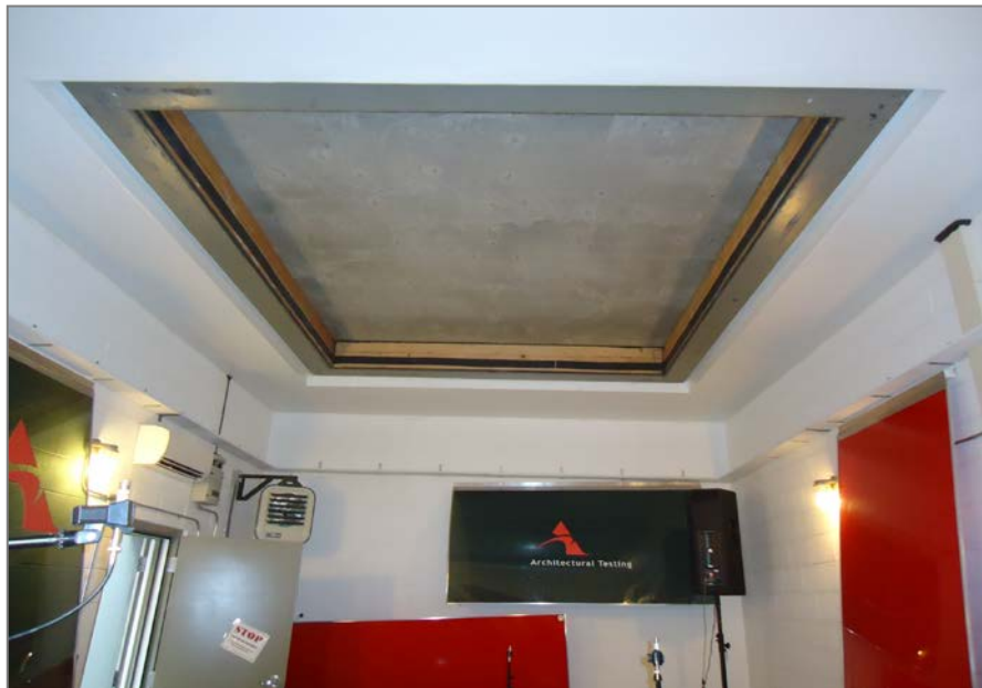
Receive Room View of Test Specimen Installation
